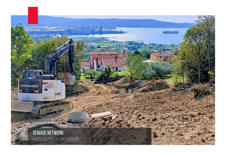
The missing part of the sewage network is being constructed in the built-up areas of Bertoki, Škofije, and Hrvatini. 14 building permits had to be obtained for the construction of 25 kilometres of sewers, 4 kilometres of drainage channels, 14 pumping stations, and a part of a replacement water supply system.
