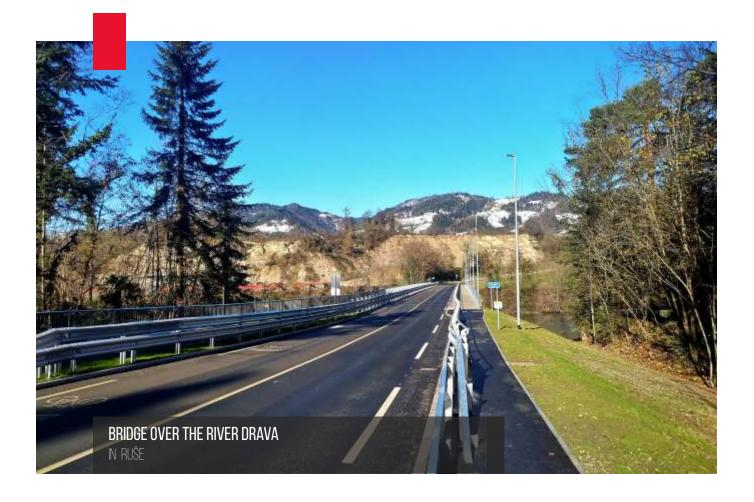
The bridge over the River Drava in Ruše, built in 1967 and renovated in 1989, required renovation due to wear and tear and new traffic conditions.
