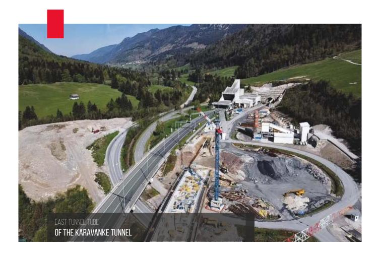
The total length of the new eastern tube of the Slovenian-Austrian Karavanke road tunnel will be 7,948 metres. Its length on the Slovenian side will be 3,546 metres, of which 3,446 metres will be underground and 100 metres will be in the form of a road tunnel gallery.
